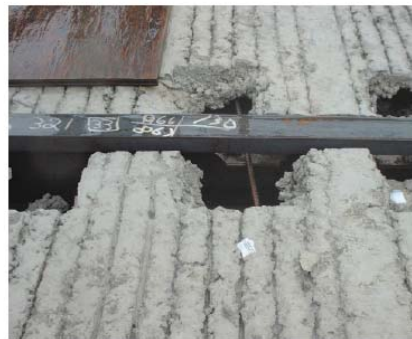
FIG 4: Floor system before topping is applied
